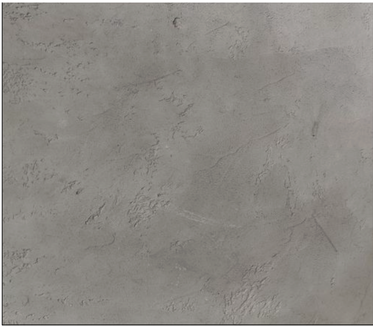
3 - LIGHT GREY CONCRETE FINISH - OFF-FORM CONCRETE
